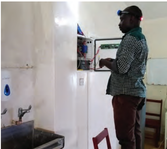
Kenyan graduate using toolkit, including headtorch, to install an MAI supplied operating light.
